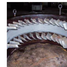
Hydro power guidevane repair
