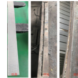
Scraper groove plate repair
