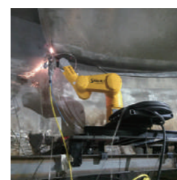
Hydro-power turbine coating
