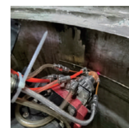
Bottom ring on-site repair
